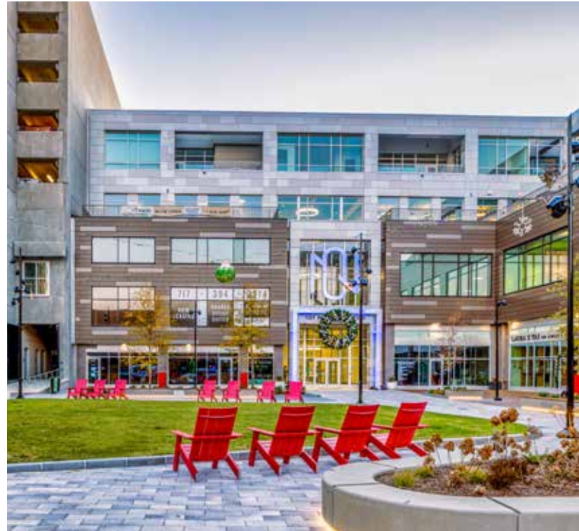
101 N. Queen is a mixed-use building complex in the Regional Commercial Hub of Downtown Lancaster City.
