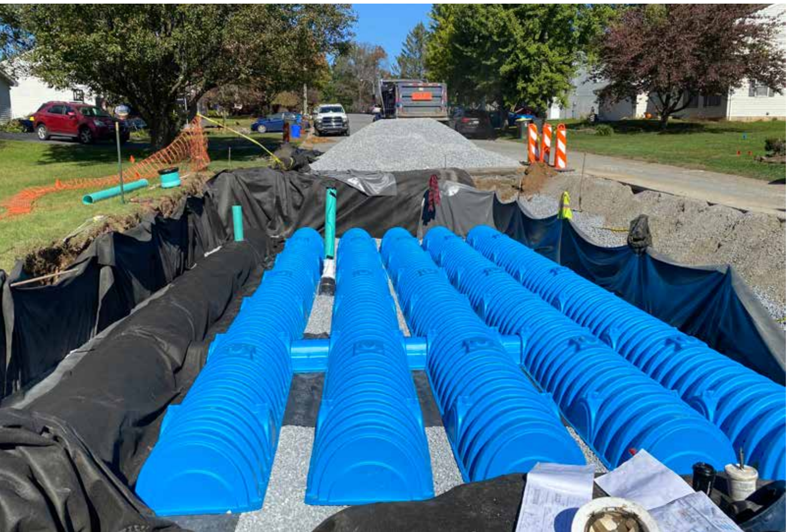
Landis Drive green storm water infrastructure installation
