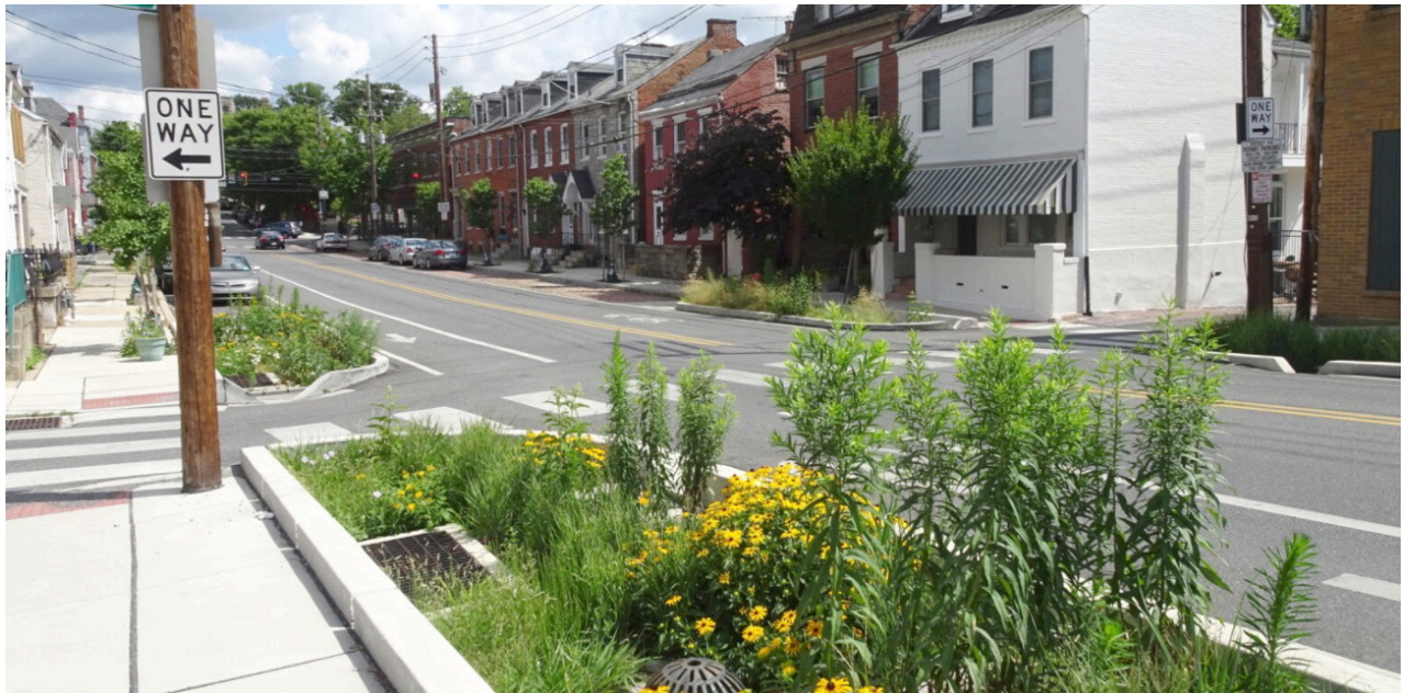
Green Infrastructure Project in Lancaster City
